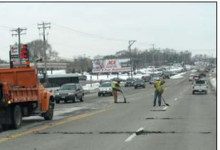
When weather allows, workers hand-apply cold patch to repair potholes in winter.
