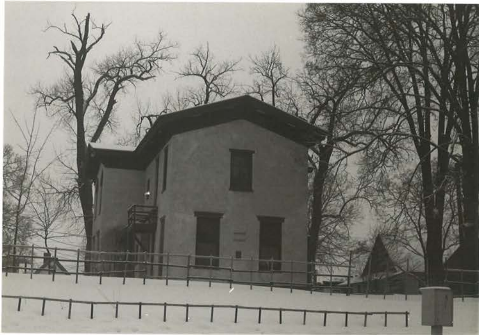
North & east facade
