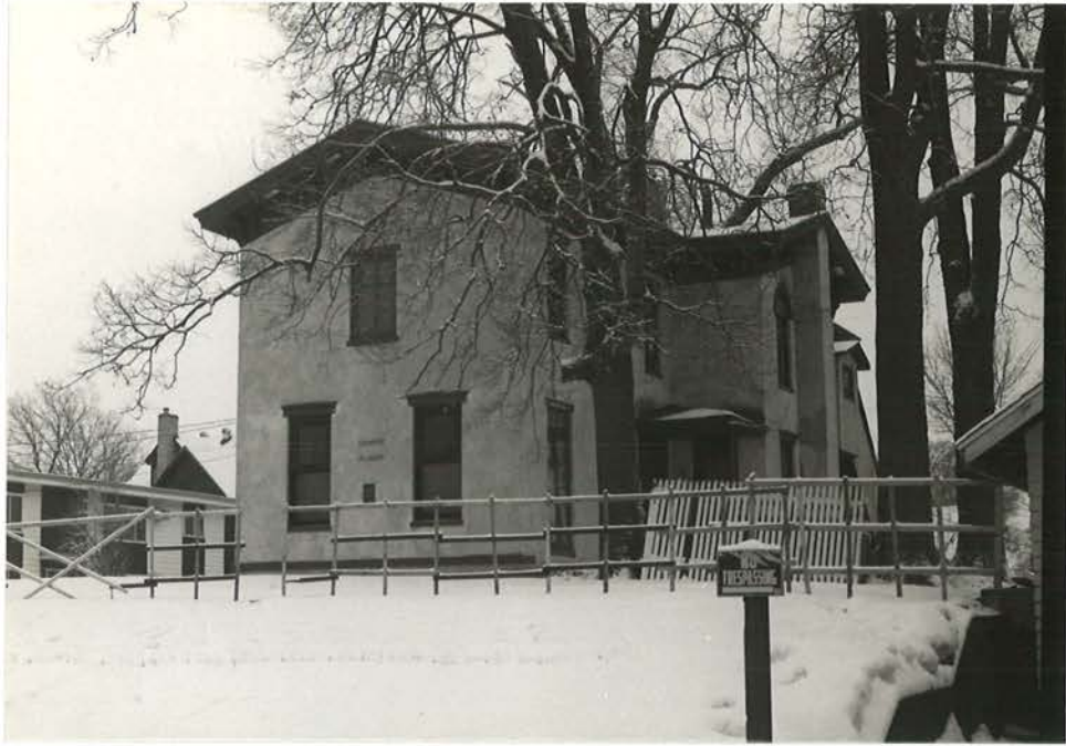
North & west facade
