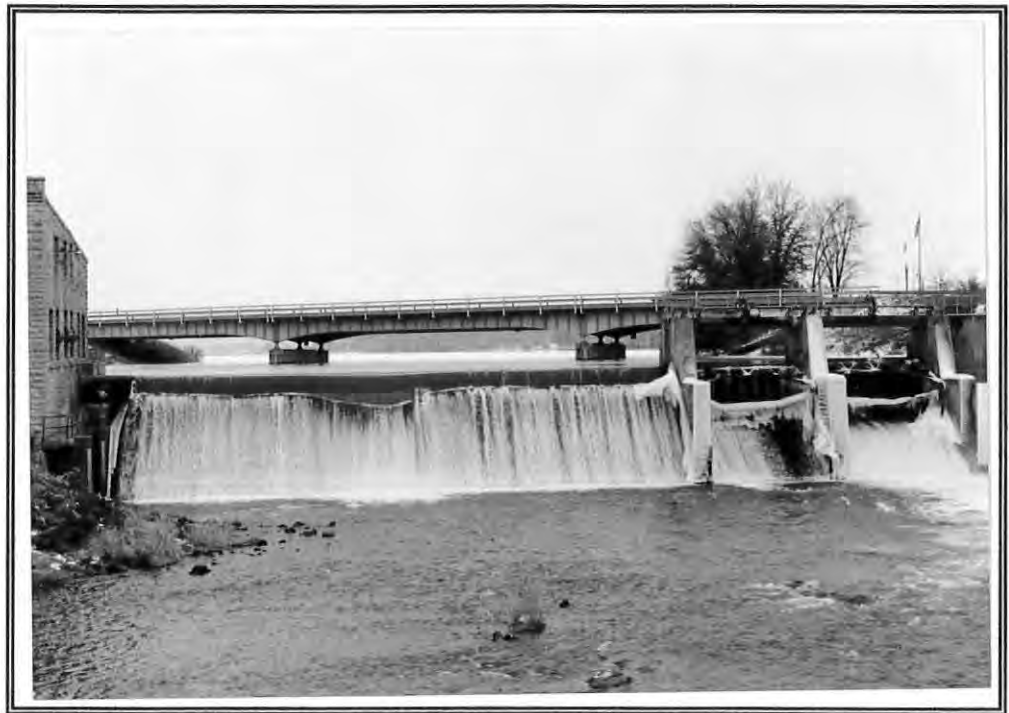
Neshonoc Dam, LC 105/09
