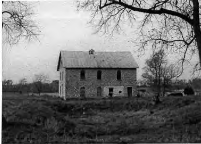
Oehler Mill (187/08), Shelby Township
