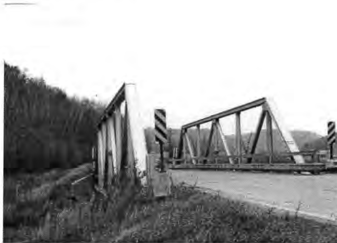
Pony Truss Bridge (190/31), Washington Township
