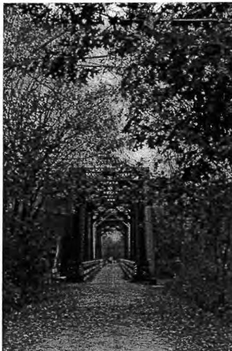
Chicago & Northwestern Railroad Bridge, Onalaska Twp., LC 207/12
