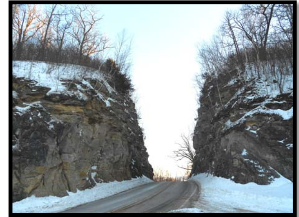
#5-Mindoro Cut* - The Mindoro Cut is located in the Town of Farmington along STH 108. This cut is the second deepest cut built by hand in the Western Hemisphere and the oldest functional cut which has not been improved upon. Work began on the cut in 1907 and it was completed in 1908.
